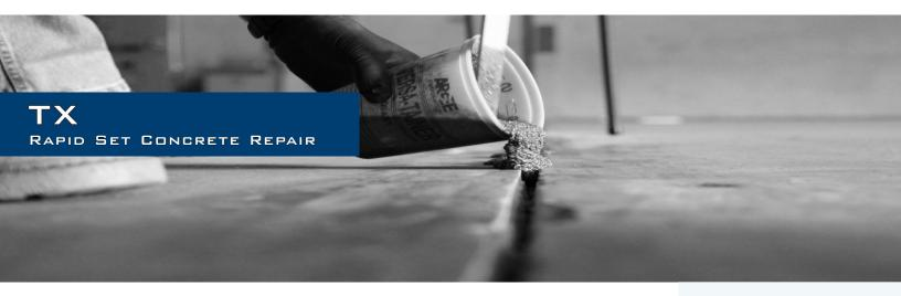
TX is a rapid set, high strength low viscosity urethane repair material. This two part, 1:1 system is 100% solids and designed for rebuilding and repairing broken control joints, filling voids under tile and concrete, and repairing spalled concrete surfaces very quickly. TX is intended for use in damaged control joints or warehouse spall damage created by forklifts or carts with steel or hard urethane wheels.
